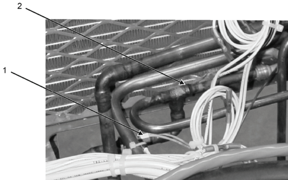
Figure 7. Condenser Coil Debraze
