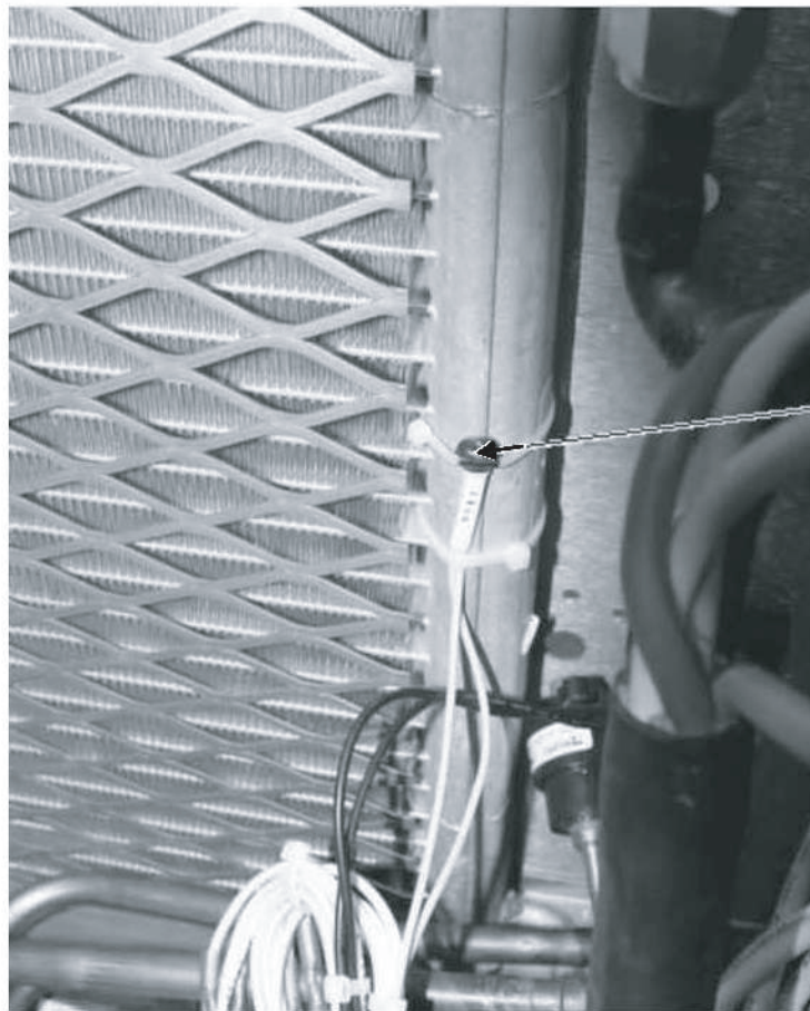
Figure 4. Location of TS5 Thermistor
